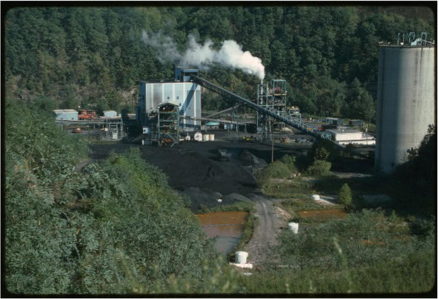
**Item Title** Coal cleaning plant as viewed from the **sludge** dam. The pond is filled with waste from the **coal cleaning** process
